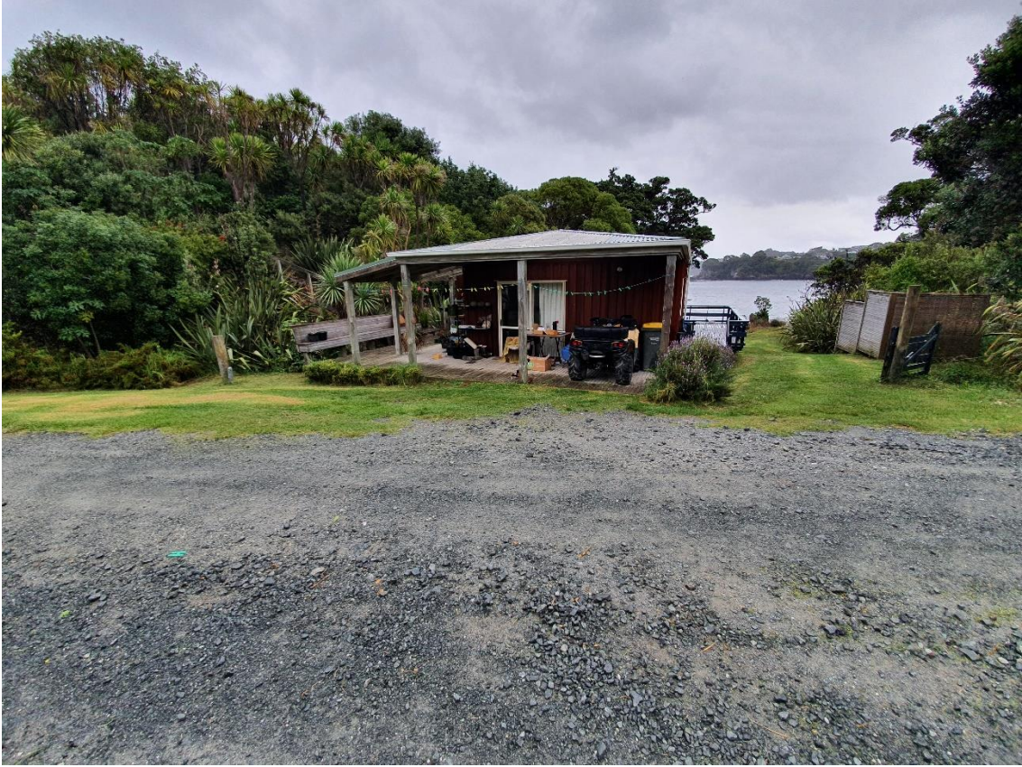
Figure 32: Looking south over Accommodation 2 site and existing dwelling.
